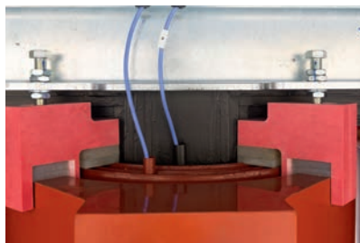
GPO3 Coil Support Blocks
