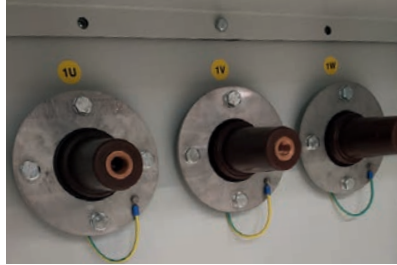
HV Cable Box with Separable Connectors
